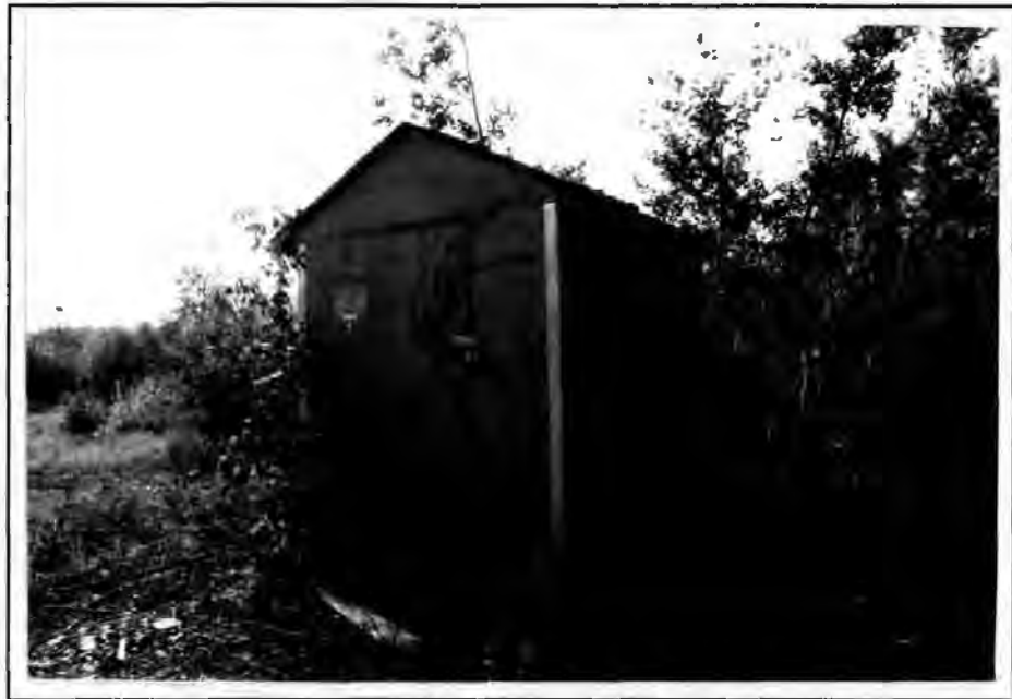
Figure 103. The BLM Airstrip Storage Building, 1993. The view is looking northeast.
